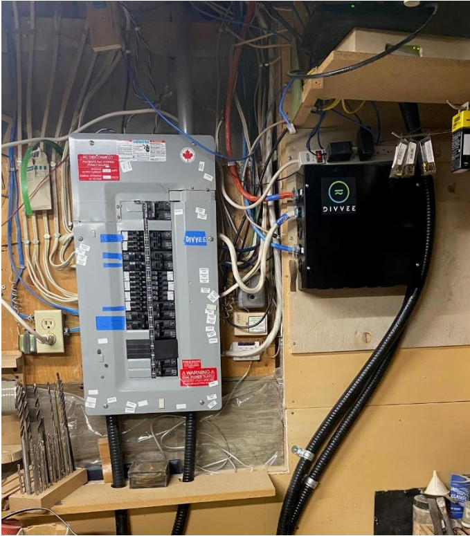
Photo: Divvee Load share device installed
