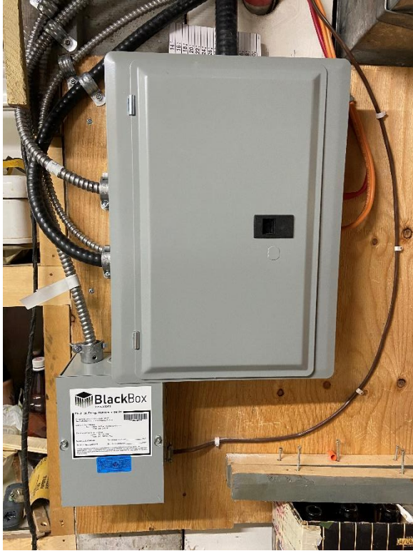
Photo: BlackBox Circuit Pauser installation
