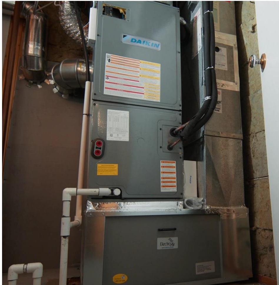
Photo: Daikin Multi-position Heat Pump Air handler indoor unit
